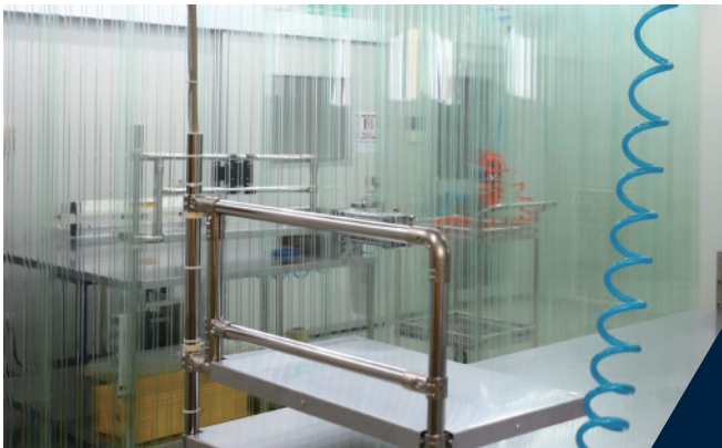
Core Competency – Sanitary Clean Room
